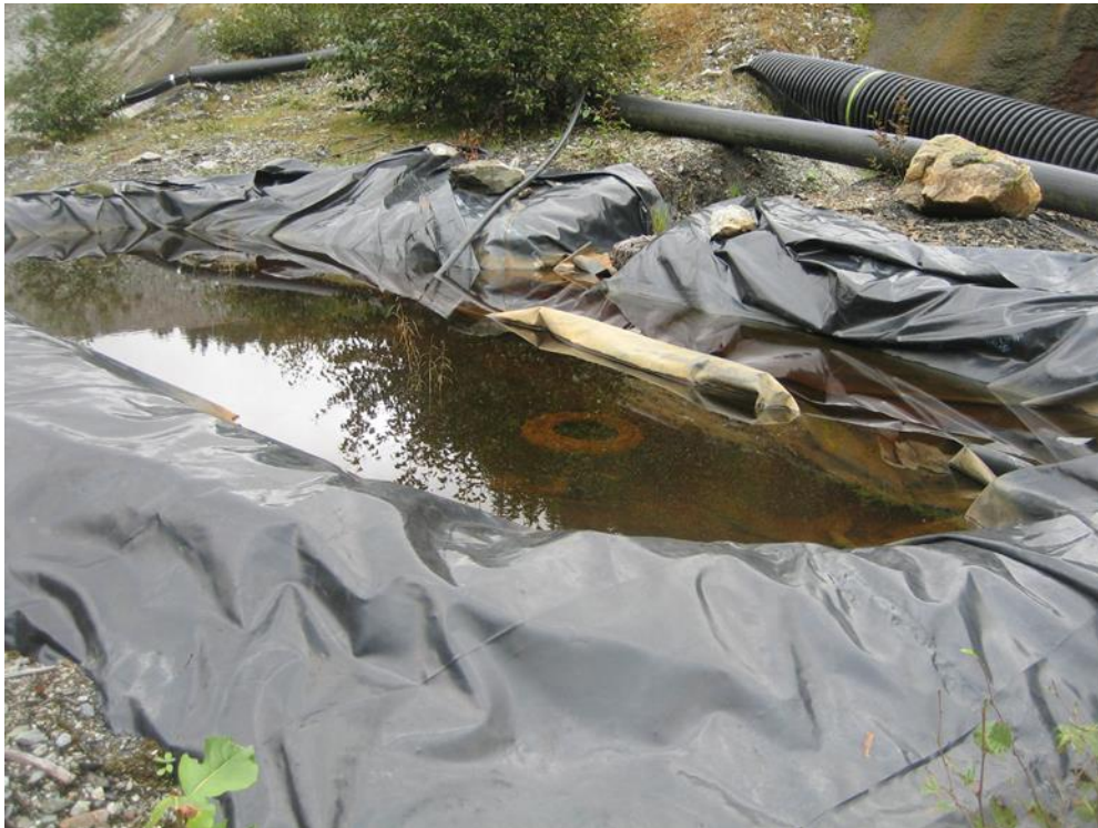
Photo HH Geomembrane-lined ARD seepage collection sump downstream of Lower Slate Lake Dam.
