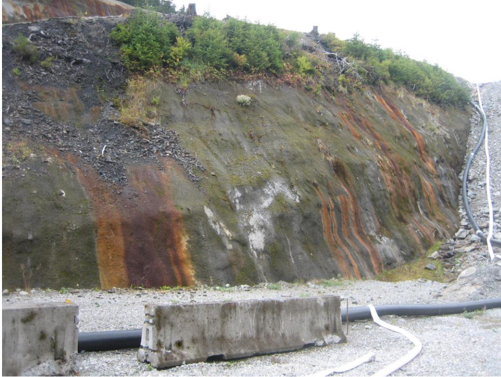
Photo CC Lower Slate Lake Dam Seepage Collection Sump return pipeline along west groin of dam. Shotcreted west abutment wall with staining from ARD seepage.
