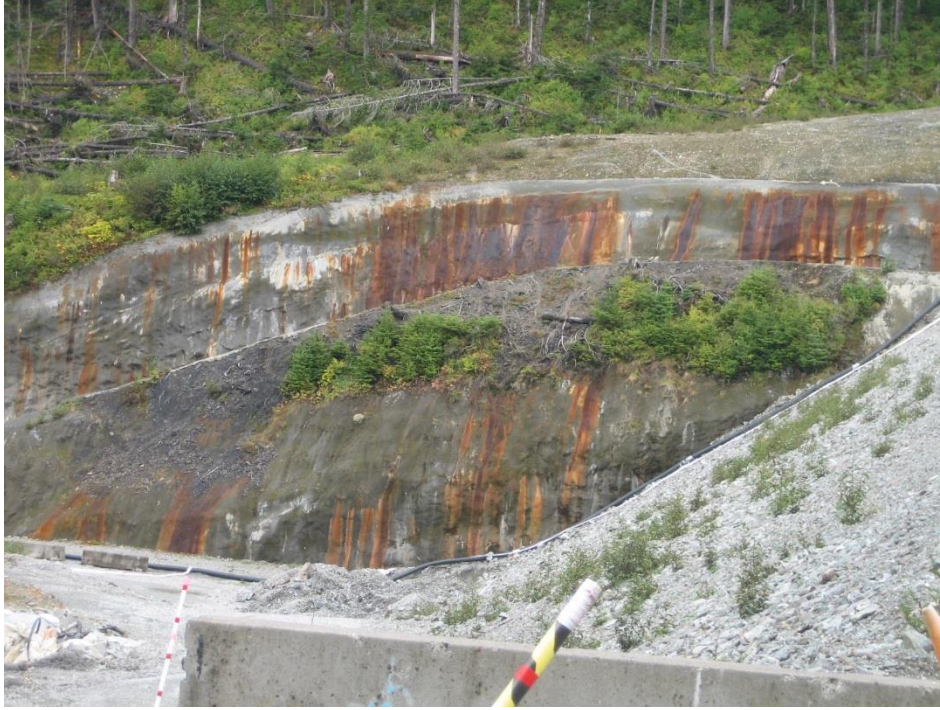
Photo Q Stage 2 Interim Spillway west wall and west abutment wall below spillway and downstream of Stage 2 Dam toe, shotcrete spillway walls with ARD seepage staining on spillway & abutment walls, looking west.
