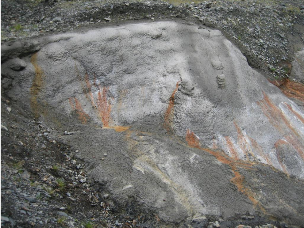
Photo T Lower Slate Lake Dam area downstream of east (left) abutment, shotcreted slopes (understood to have been excavated to rock) with staining from ARD seepage and collected seepage at toe of slope.
