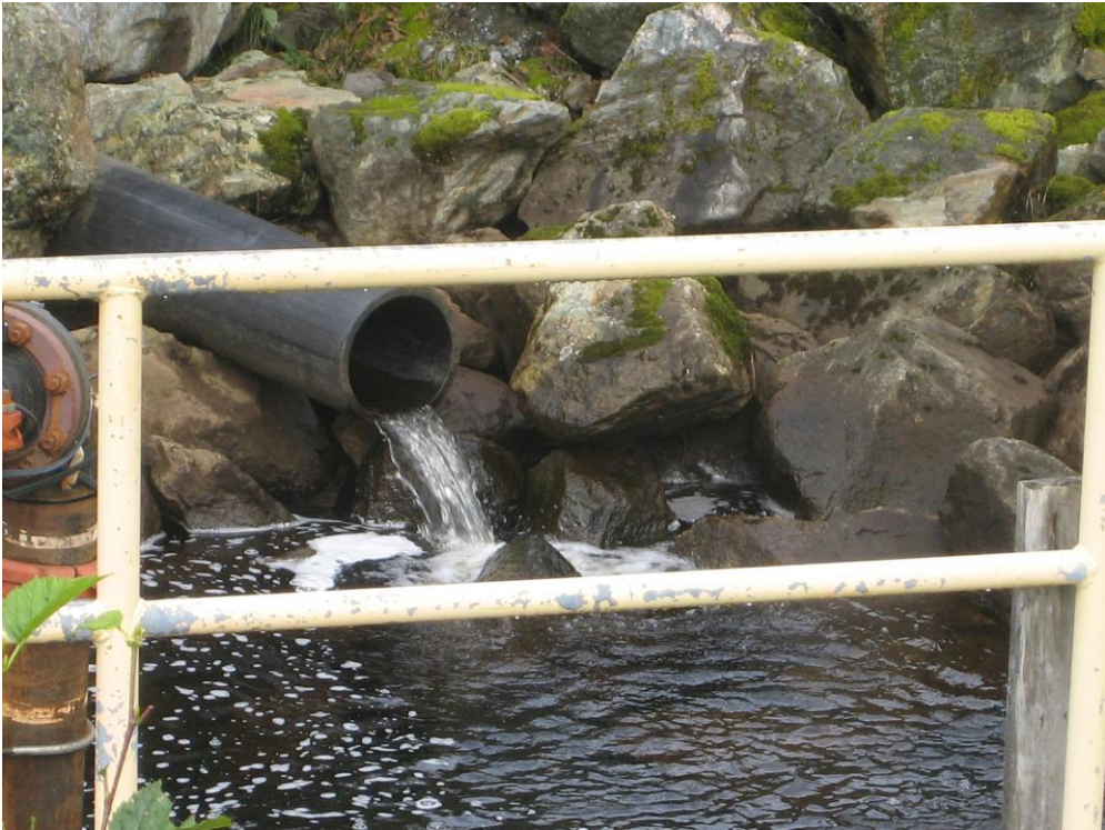
Photo D Upper Slate Creek Diversion Dam
