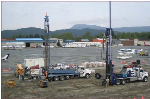
Figure 1. Vertical borings for JNU Airport loop field. Image courtesy of JNU staff
