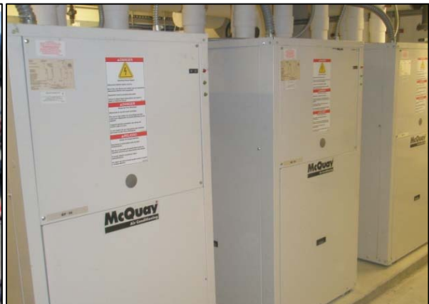
Left: Drilling for ground loop at the Juneau Airport. Right: Water-to-water heat pumps.
