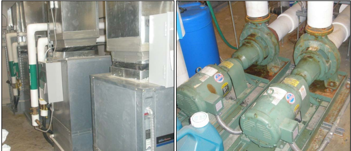
Left: Water-to-air heat pump units in the attic. Right: Circulating pumps.
