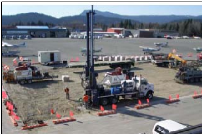
Left: Drilling for ground loop at the Juneau Airport. Right: Water-to-water heat pumps.
