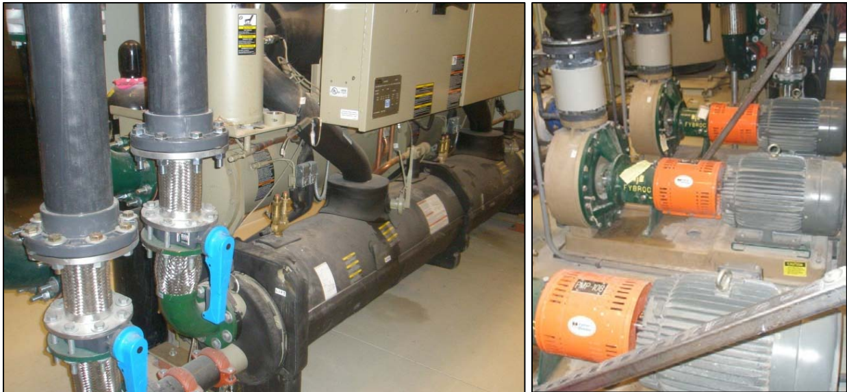
Left: Water-to-water heat exchanger. Right: Seawater treatment pumps.
