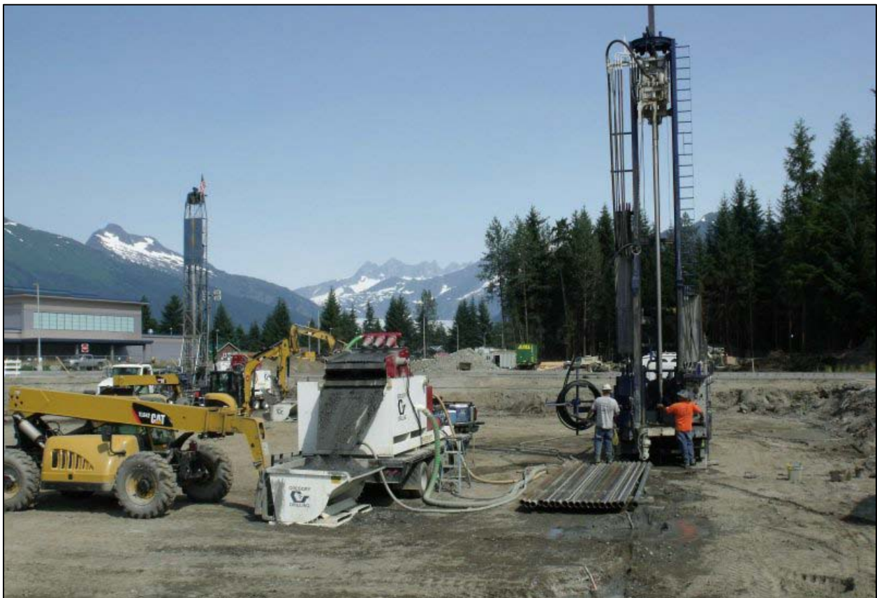
Above: Drilling at the Dimond Park Aquatic Center
