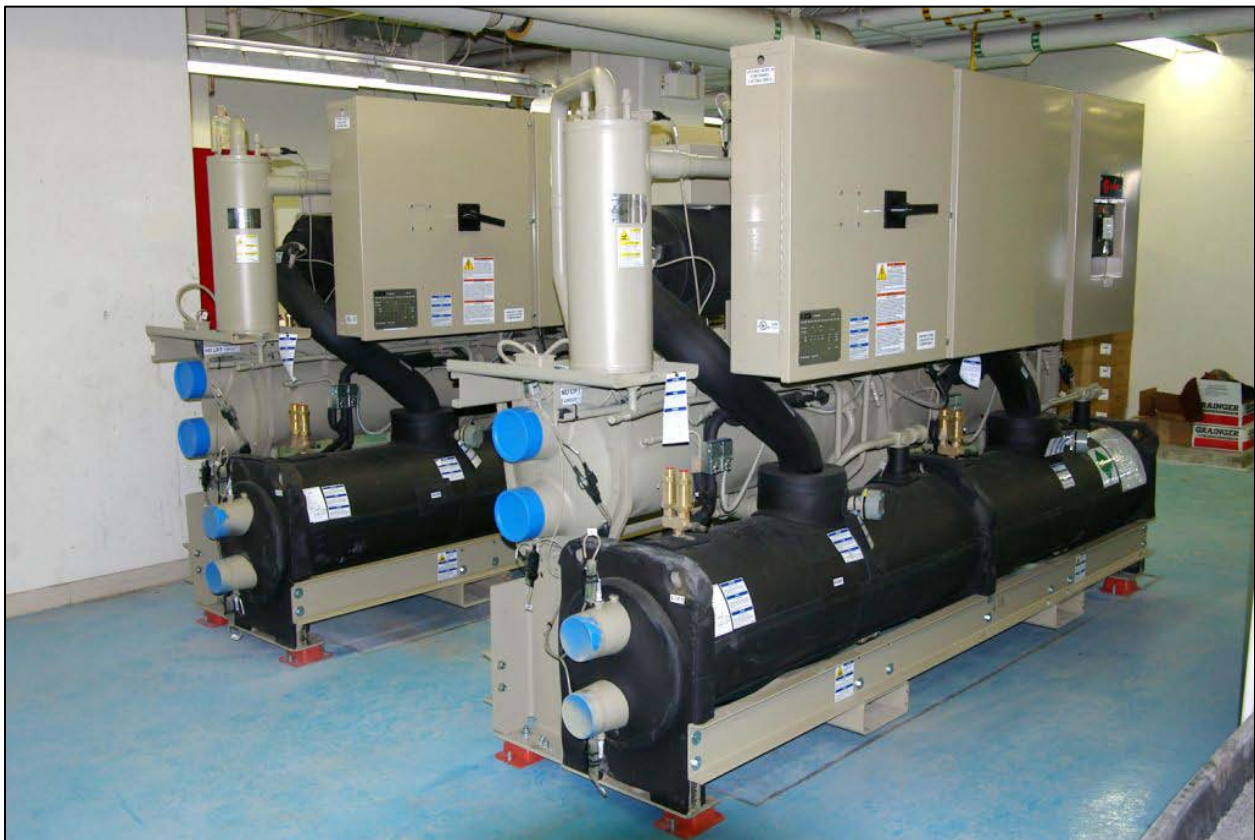
Above: Heat pump units installed and ready for connections, 3-18-11
