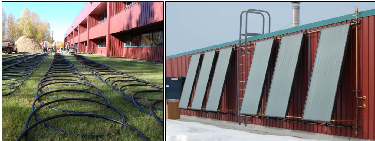
Left: Preparation of “slinky” ground loops. Right: Solar thermal collectors for hybrid GSHP.
