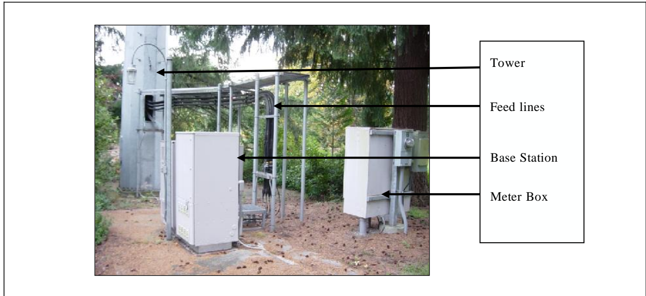
Figure 1: Example of 1900 MHz Wireless Infrastructure Ground Equipment
