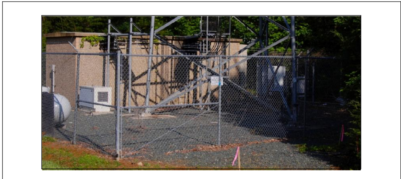
Figure 2: Example of 800 MHz Base Station
