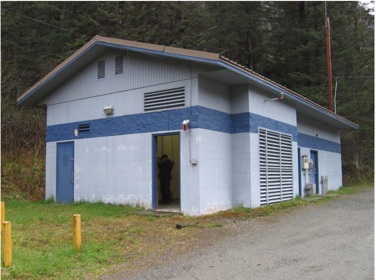
Last Chance Basin Water Treatment Building (Gold Creek)#
