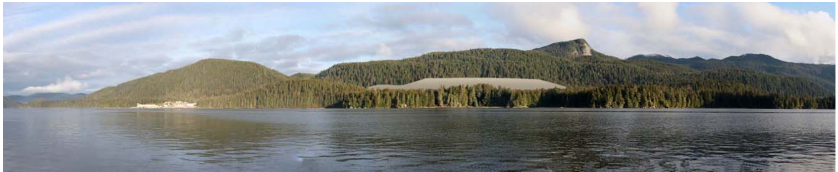
Figure 3.14-6. Alternative B: Photo-Simulation from Hawk Inlet showing Alternative B TDF Expansion at Maximum Height before Revegetation.
