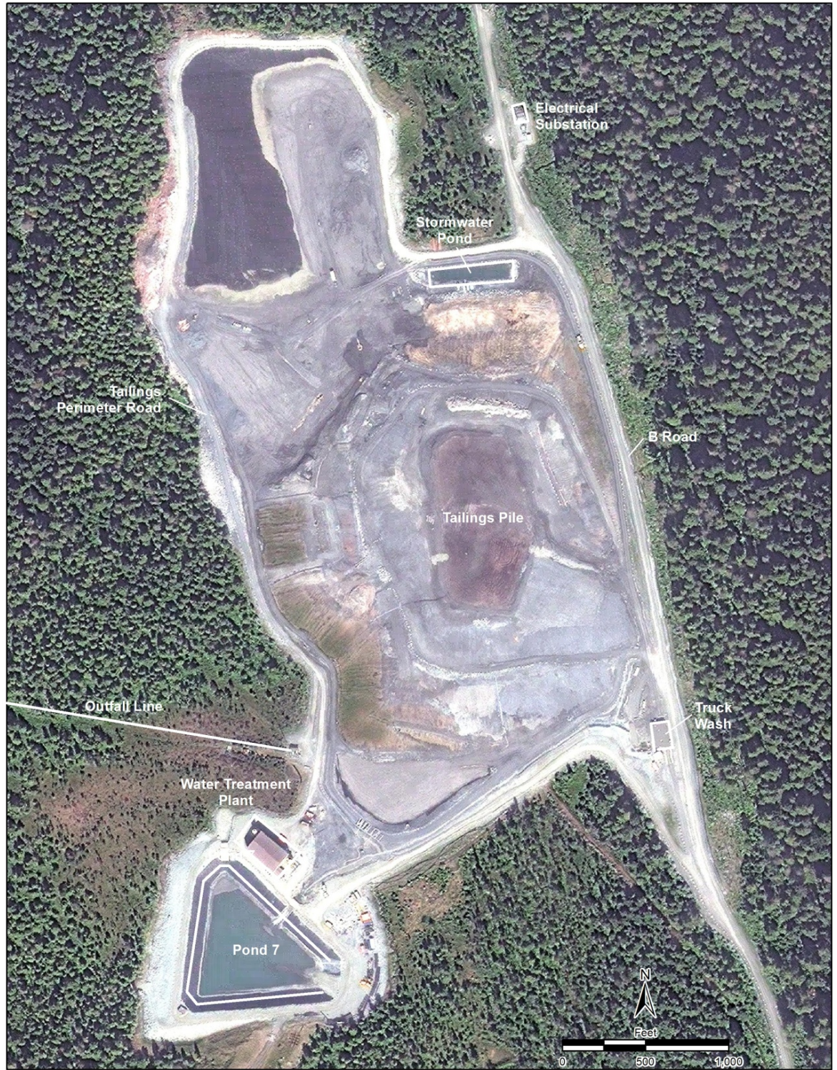
Figure 1.1-3. Greens Creek Tailings Facility.
