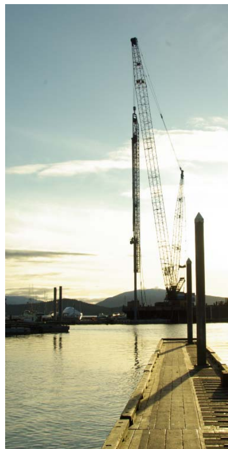
Construction in Statter Harbor (Photo Credit: Andy Wink).
