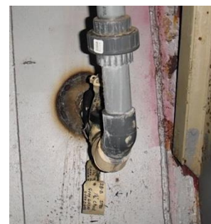
Figure 2 Direct Grey Water Overboard Discharge Port
