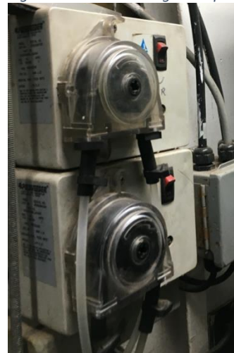
Figure 7 Chlorine Dosage Pumps
