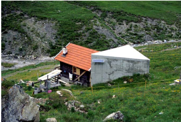
Fig. 35: Avalanche wedge made of concrete to protect an endangered building on an alp (Switzerland). The wedge was built some years after the construction of the hut.
