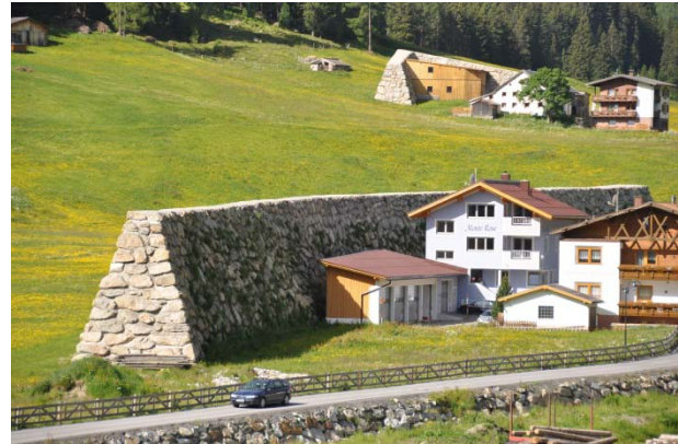
Fig. 36: 10 m high wall for the protection of buildings in Galtür (Austria). The wall was built some years after the construction of the buildings.
