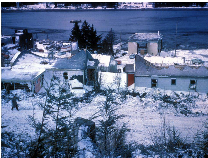
Fig. 15: View of Behrends Avenue with Gastineau Channel in the background – collapsed roofs due to overpressure and impacts of trees. The back-walls are not damaged.
