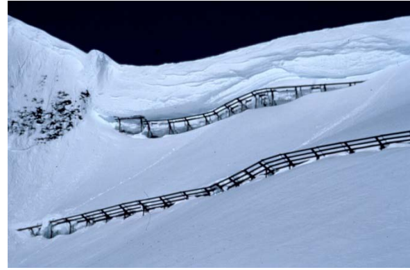
Fig. 30: The structure height is decisive for their effectiveness and for the structural design. Overfilled structures can be damaged and avalanches can break loose above the structures.
