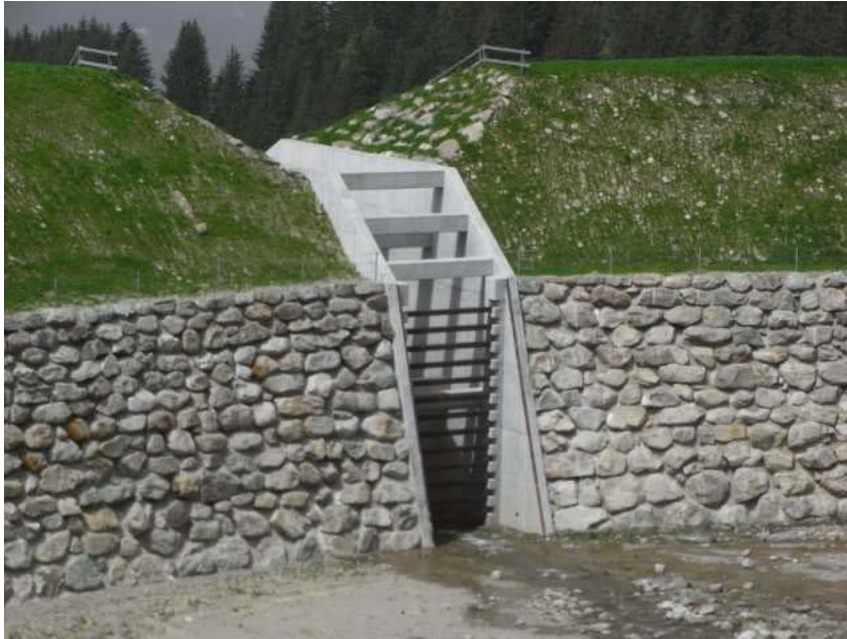
Fig. 51: Example of a combined avalanche/debris flow catching dam (view downstream). The height of the dam is 17 m. The dam is designed to stop a 30-year avalanche (Tallawine, Klosters, Switzerland).
