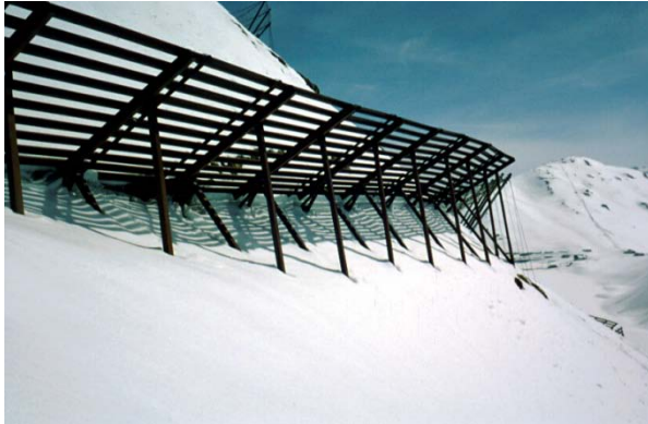
Fig. 29: Snow supporting structures in the Swiss Alps. The structures consist of snow bridges made of prefabricated steel elements.
