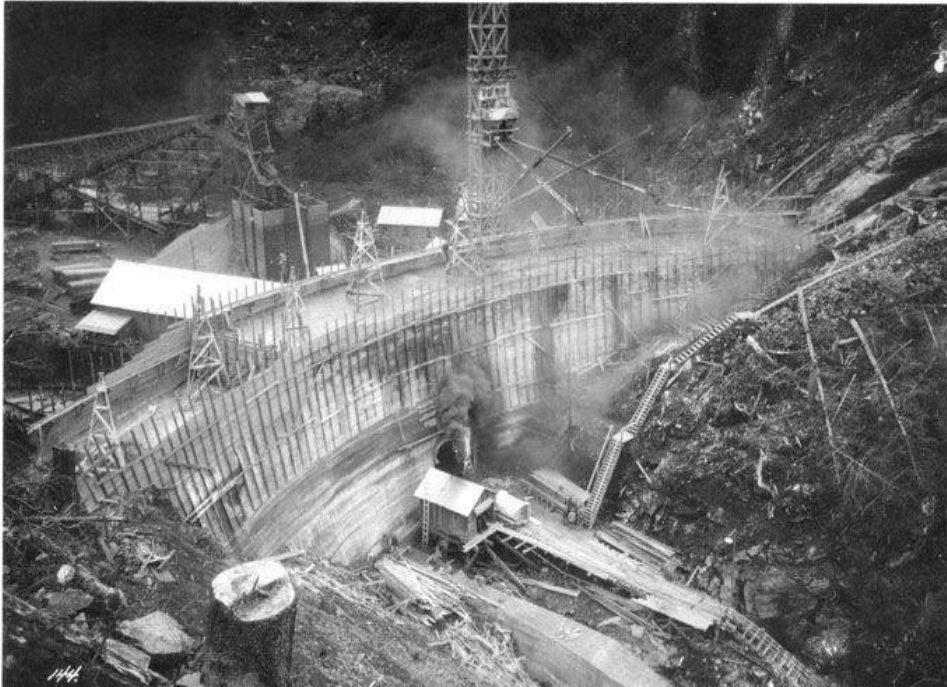
Figure 14. Salmon Creek Dam under construction c. 1913-1914 (photo: Alaska State Library ASL-M999-AEL&P-144WP).
