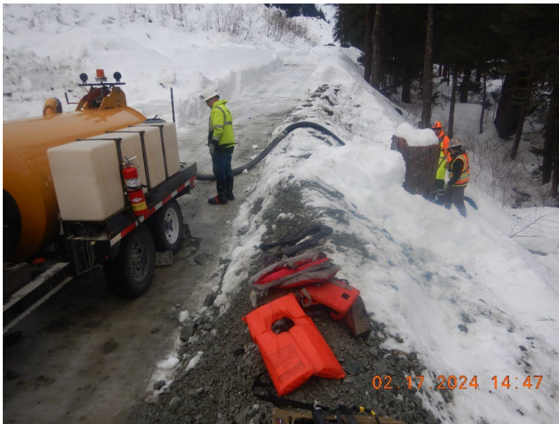
Photo 5. Vacuum trailer removing tailings near Johnson Creek.
