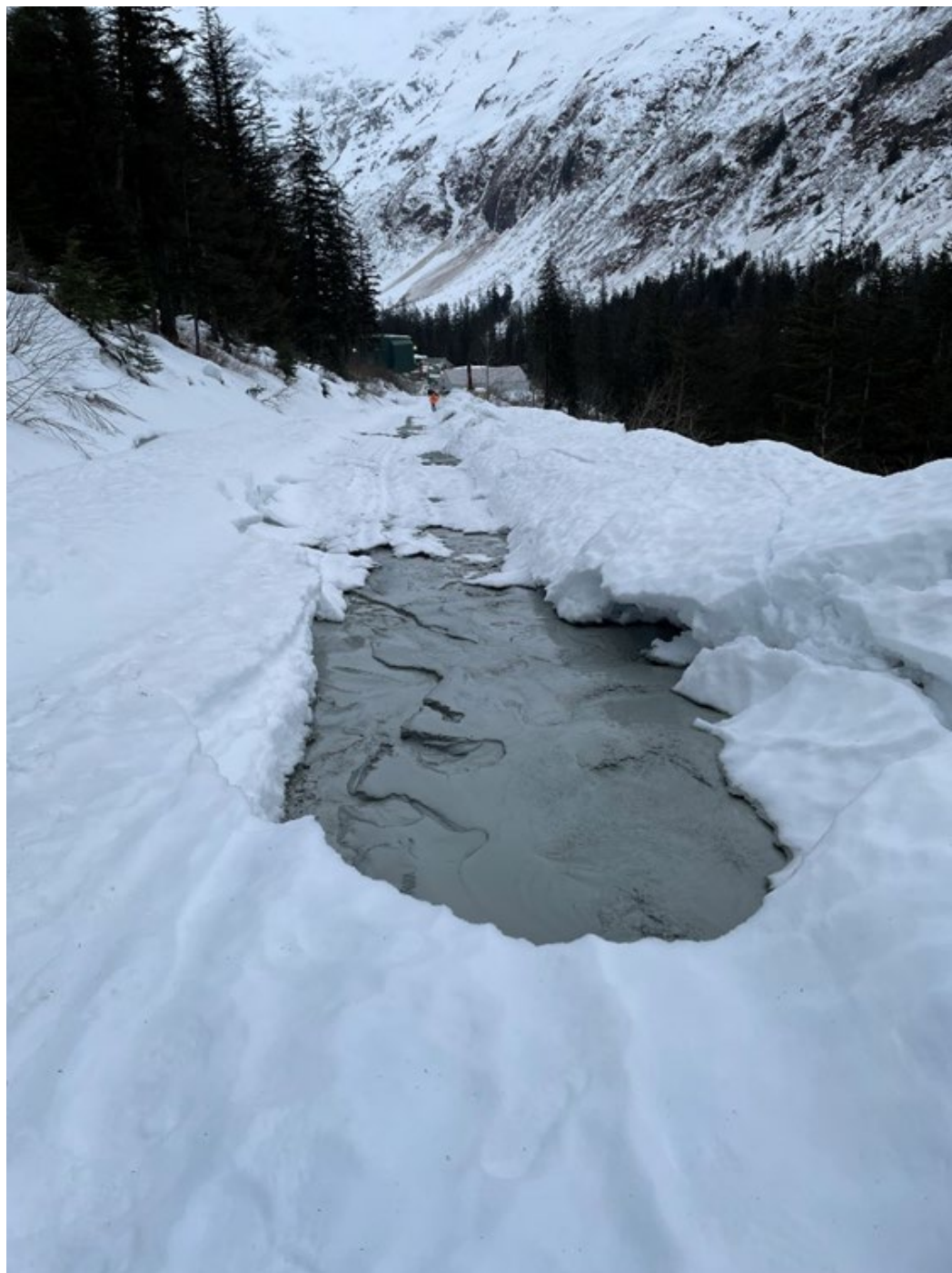
Photo 1: Tailings leak from buried tailings line on Pipeline Rd.
