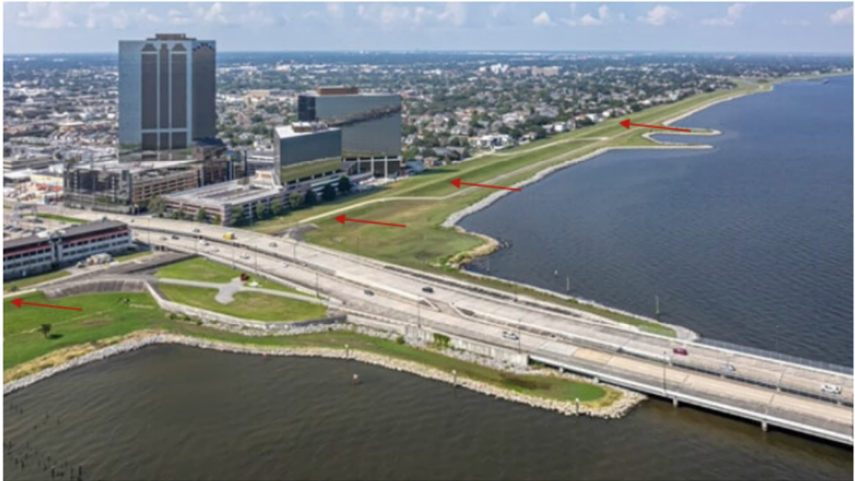
Figure 4-20 Levees Protecting Suburban Neighborhood with Over-Top Roadway Crossing
