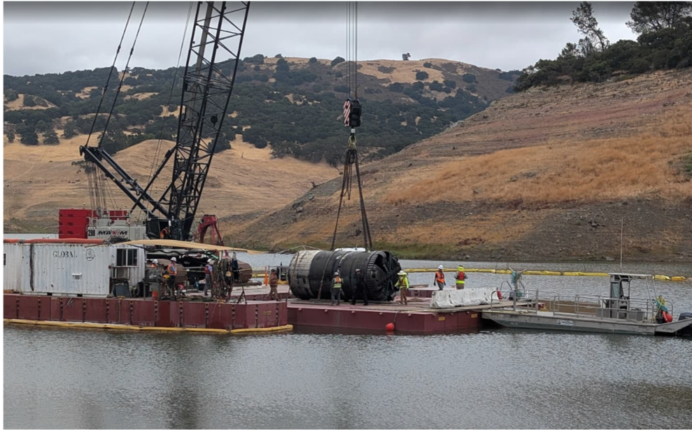
Figure 4-6 8-Foot-Diameter Micro-Tunnel Boring Machine Being Recovered
