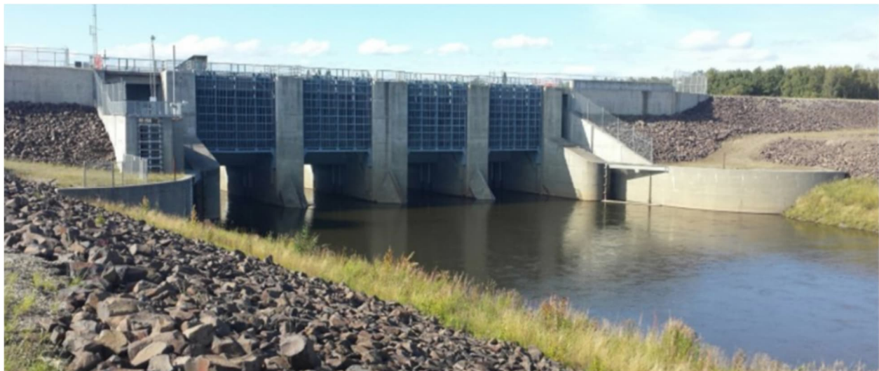
Figure 4-18 Outlet Works from Moose Creek Dam
