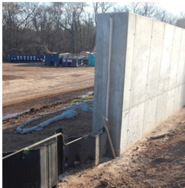
Figure 4-24 Photo of I-Wall in Construction
