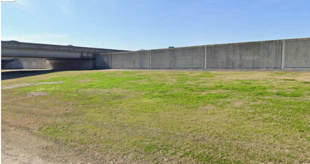
Figure 4-27 T-Wall Photograph – Interstate Bridge Crossing through a Flood Protection System
