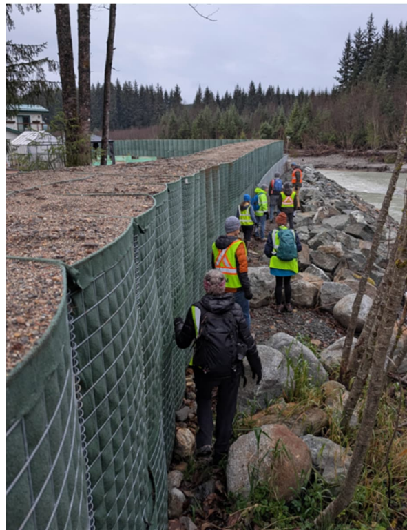
Figure 4-46 Current 8-Foot-Tall HESCO Barrier Near Melvin Park; Proposed Floodwalls Would Likely Average Approximately Double the Height of These Barriers
