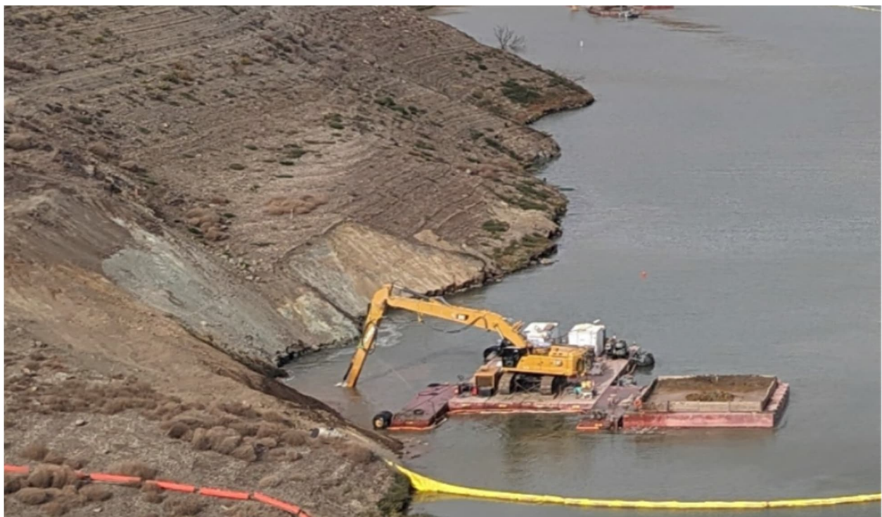
Figure 4-7 Long-Reach Excavator and Spoils Barge Performing Dredging on Lake
