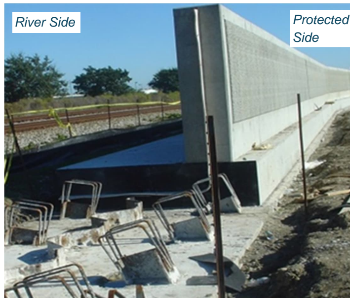
Figure 4-26 T-Wall Photograph – Cross-Section During Construction
