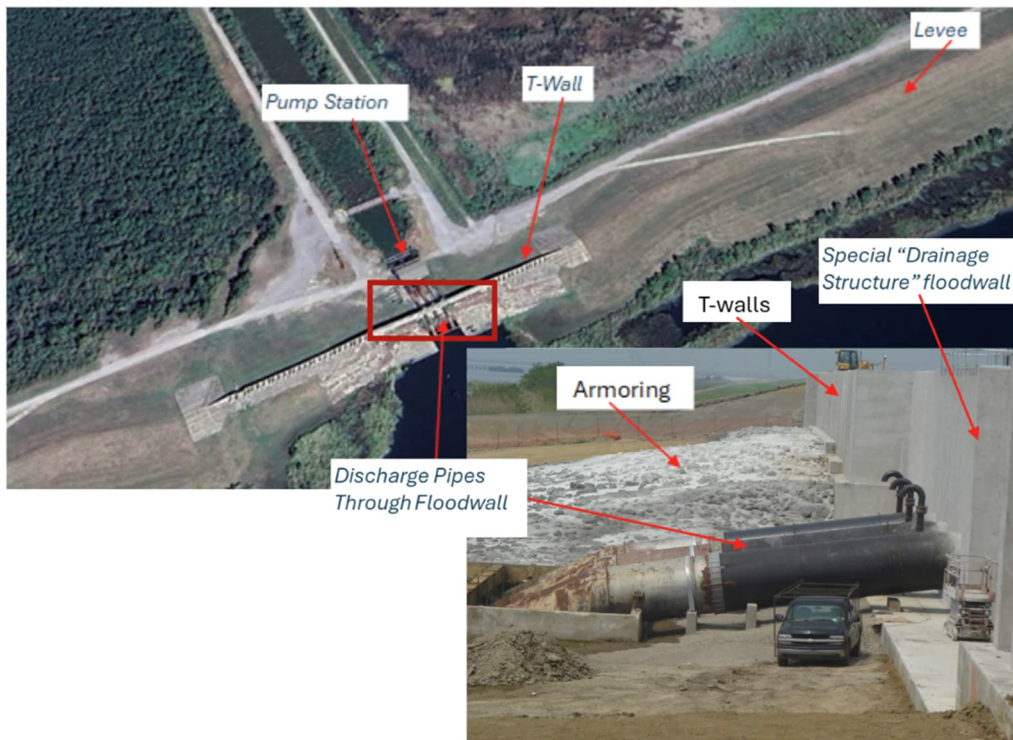
Figure 4-32 Typical Pump Station and Associated Discharge Piping Arrangement in FRMS (View Is of Protected Side Wall Face)
