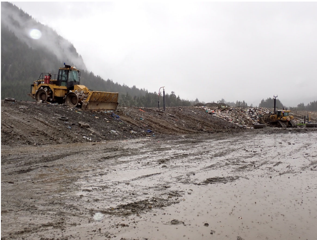
Figure 14. Well covered and compacted waste near the active face of the landfill.
