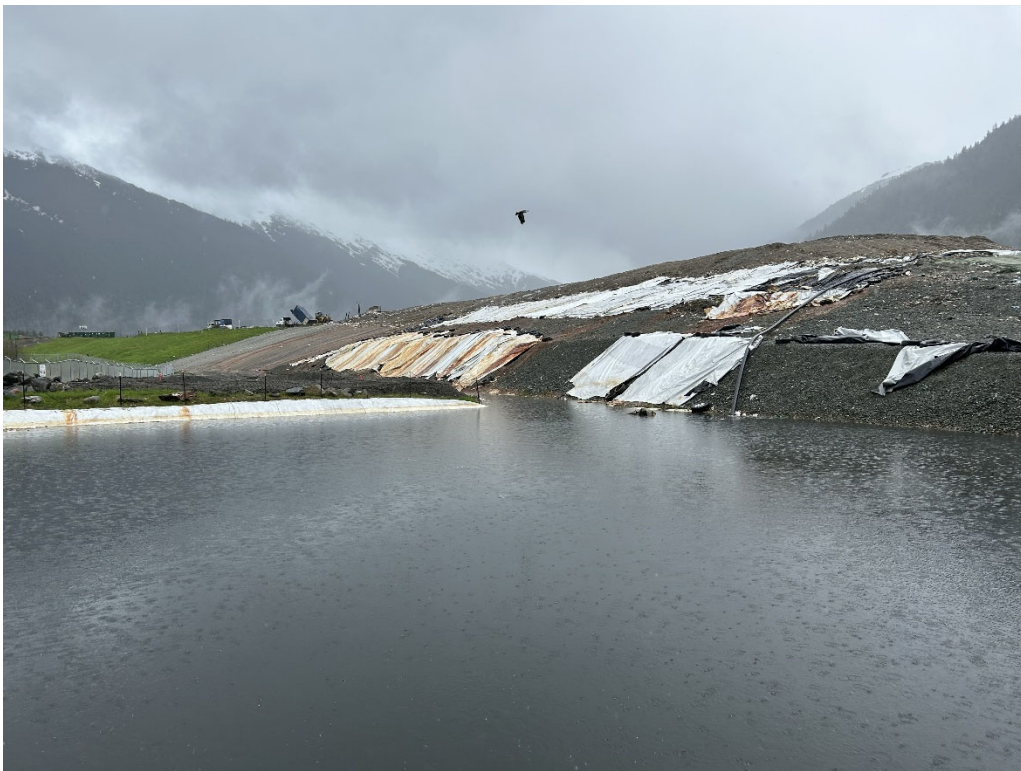
Figure 8. Leachate detention pond with landfill in background including historic waste in the background with grass, waste covered with a synthetic intermediate cover system, and some waste covered with daily plastic cover and earth.
