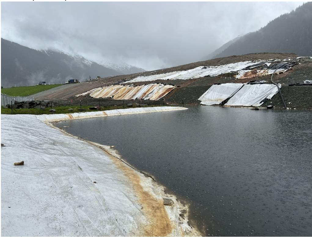
Figure 5. The leachate detention pond in the southwest of the facility is lined.
