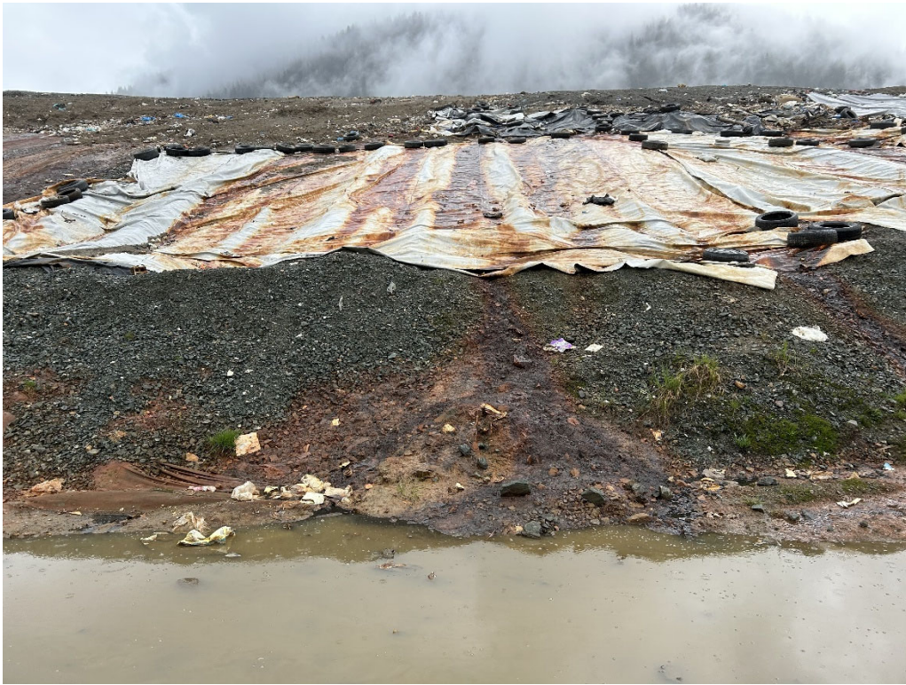
Figure 11. Leachate seeps from the active area of the facility flowing directly into the stormwater system.
