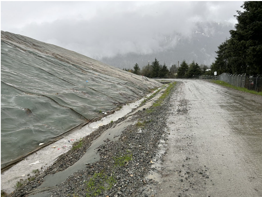
Figure 2. The northeast portion of the landfill has synthetic intermediate cover that appears to be functioning well in heavy rain.
