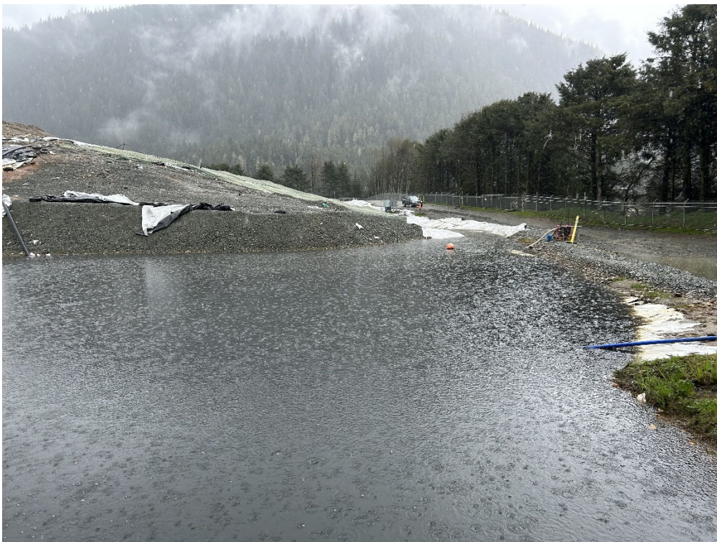
Figure 6. The leachate detention pond in the southwest of the facility has a level that overtopped the liner.
